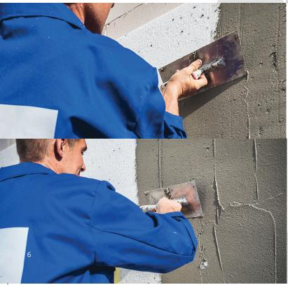
Apply the ready plaster/adhesive mass in a continuous layer, approx. 3-4 mm thick.
